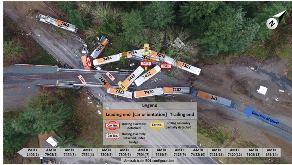
Figure 3 – Annotated aerial view of Dupont, WA, derailment scene captured by Washington State Police helicopter (National Transportation Safety Board 2019)
