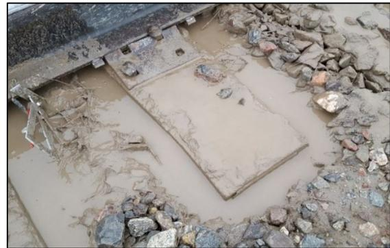
**Figure 1. Photograph of mud pumping with standing water**
